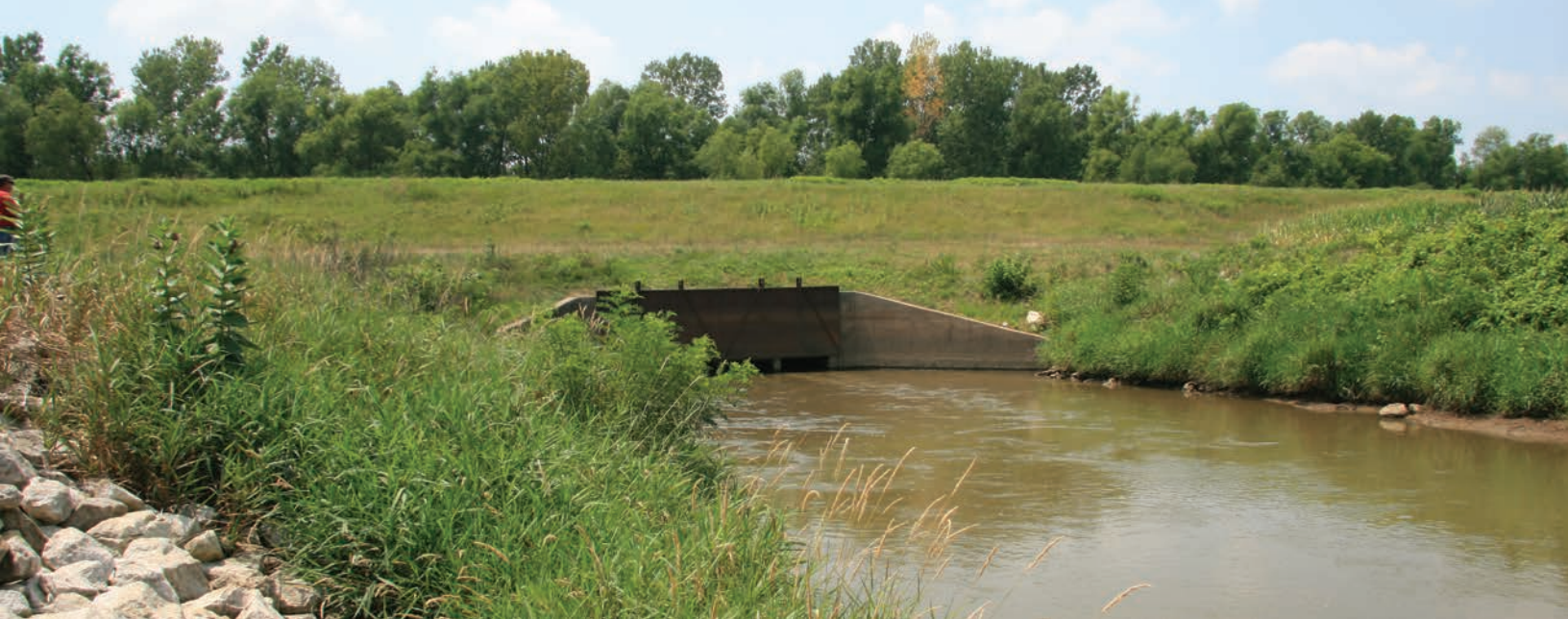
FIGURE 1.3 One of two Sny River aqueducts transports floodwaters and sediment to settling basins.
