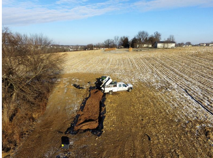
Bioreactor installation in Polk County, Iowa. SWCS/IDALS photo by Lynn Betts.
