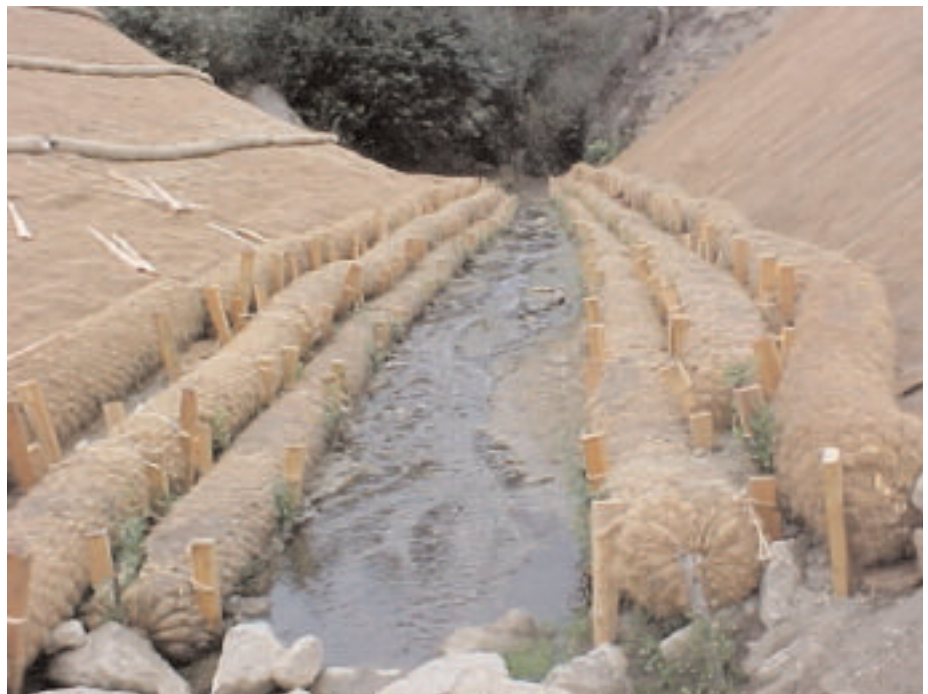
Figure 2. Densely-packed coir logs placed on a stream.
