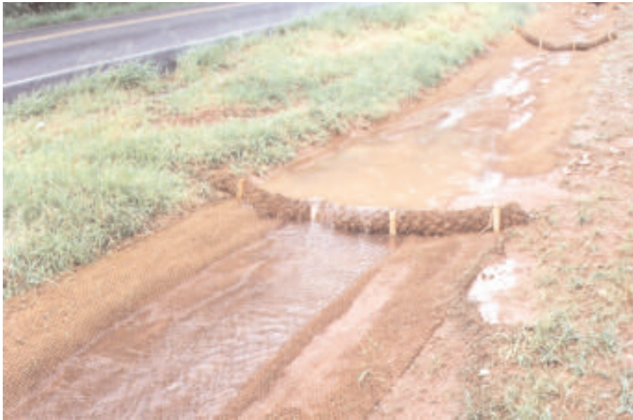
Figure 9. Vegetated waterway construction with woven coir mats and coir wattles.
