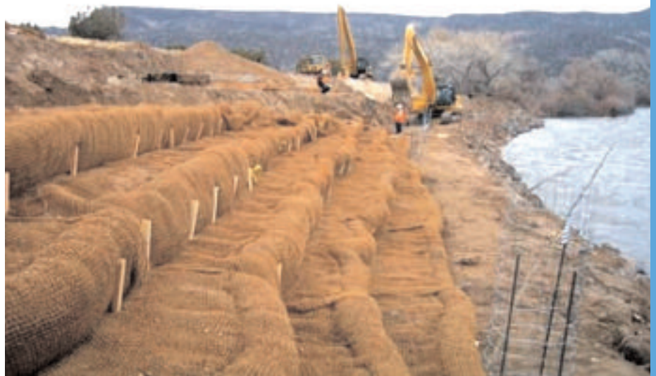
Figure 6. Soil lift construction with coir block system.
